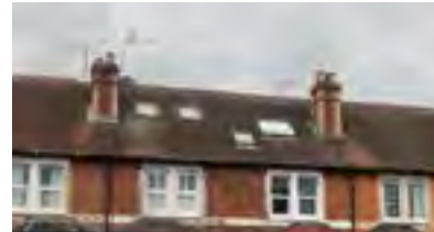
Gable roof with chimney stacks and rooflights
