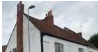
Gabled roof decorated with chimney stacks
