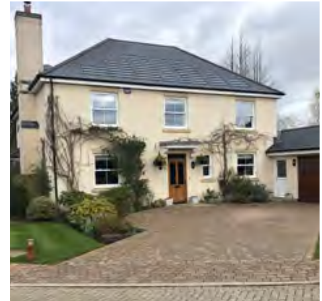
Figure 126: Use of shingle-like solar panels on a slate roof, with the design and colour of the solar panels matching those of the adjacent slate tiles.
