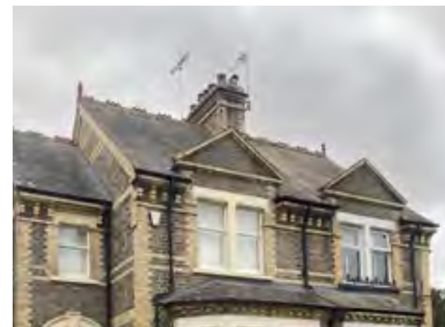
Figure 114: Local example, within the Station conservation area, of grey slate tiles on a gable roof with chimney.
