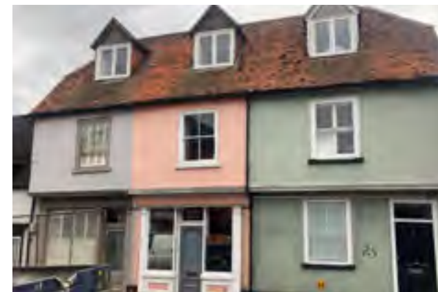
Figure 113: Local example, within the Twyford village conservation area, of clay tiles on a mansard roof with gable dormers.
