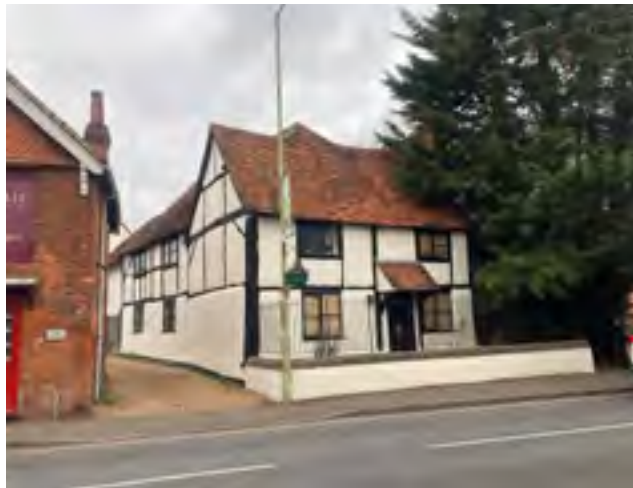
Figure 07: Old Farm House, 24 High Street (Twyford Conservation Area).
