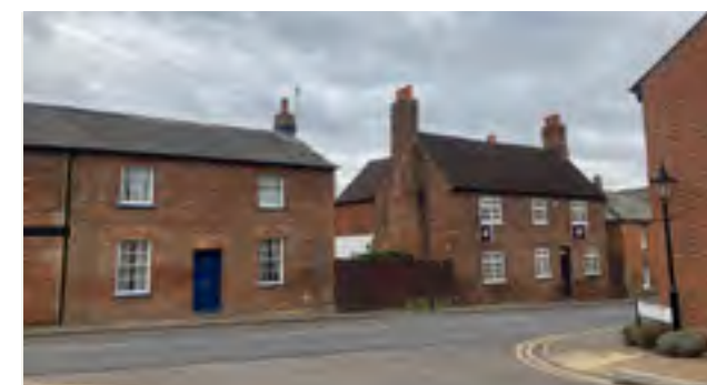
Figure 53: The recent development to the western border of the conservation area respects the opposite buildings across the street by retaining a similar scale, massing and materiality.
