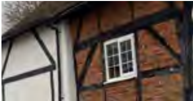
Half timbering technique infilled with red brick
