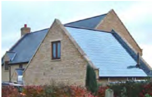
Figure 127: Positive example of implementing solar panels since the design stage.
