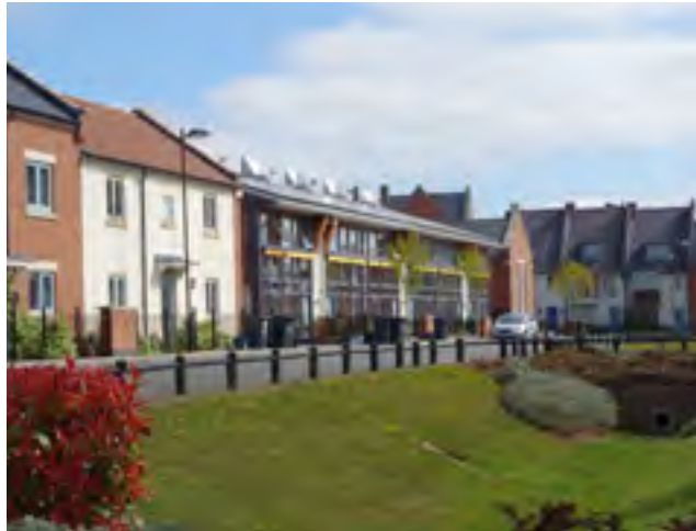
Figure 89: An example of a SuDS corridor - Upton Urban Extension, Northampton.
