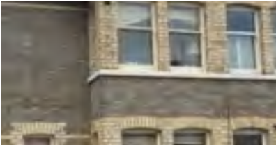
Grey brick combined with yellow brick around the openings
