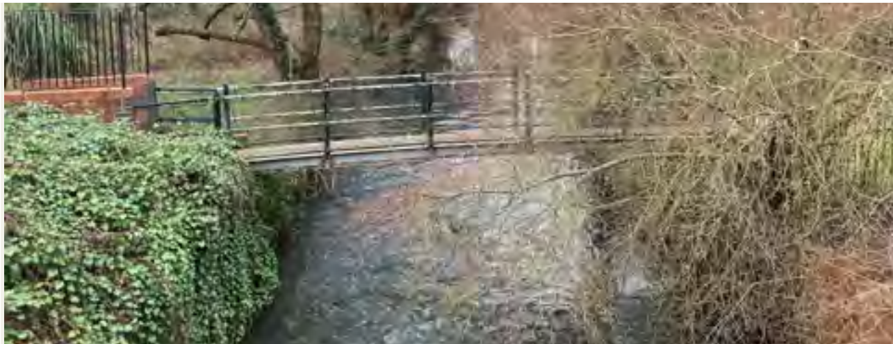
Figure 20: Footbridge providing crossing over River Loddon at Silk Lane.
