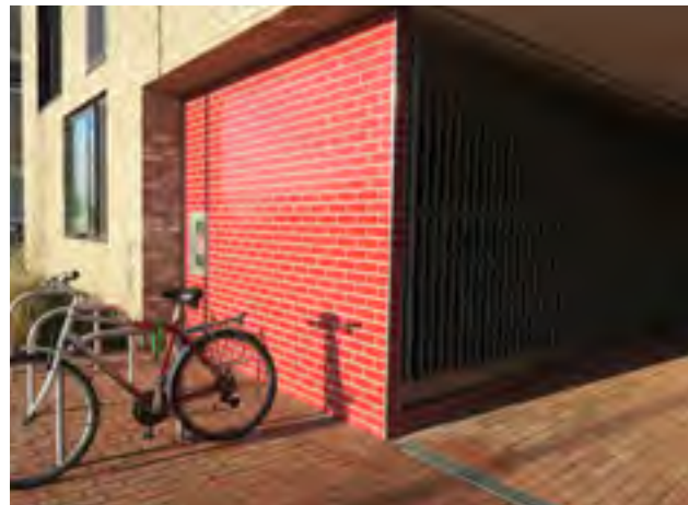
Figure 85: Example of cycle parking for houses without garages, Cambridge.
